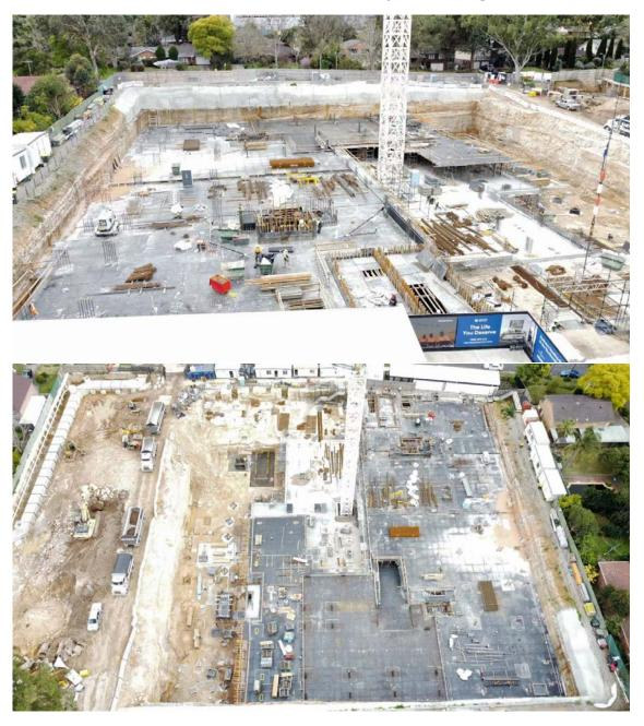
Approximately 85% of the basement excavation is completed with over 38,000 cubic metres of materials removed from the site.
